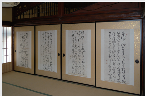
Antechamber (after repairs)
