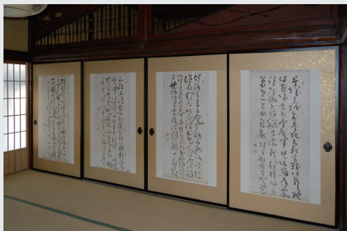
Antechamber (after repairs)
